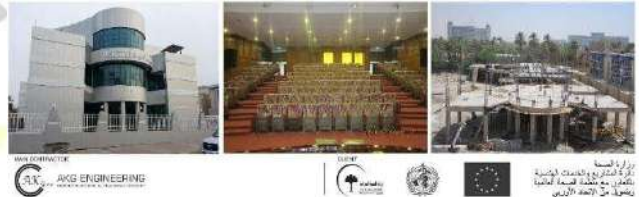
Disaster Emergency Readiness Training Center Baghdad - Completed
