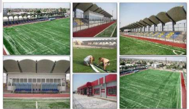
Establishment of 3 artificial grass playground – Completed
