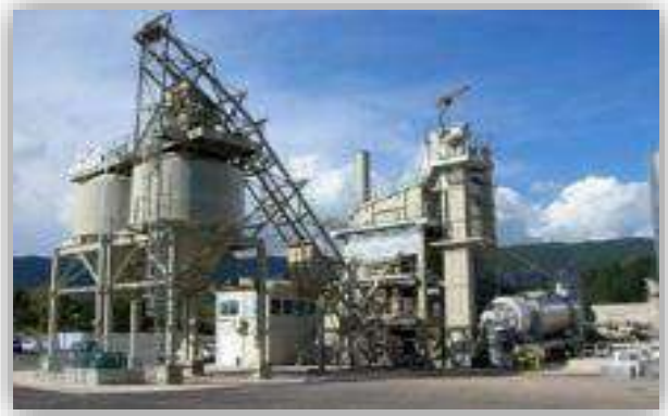
Diwaniyah Asphalt Plants –Completed
